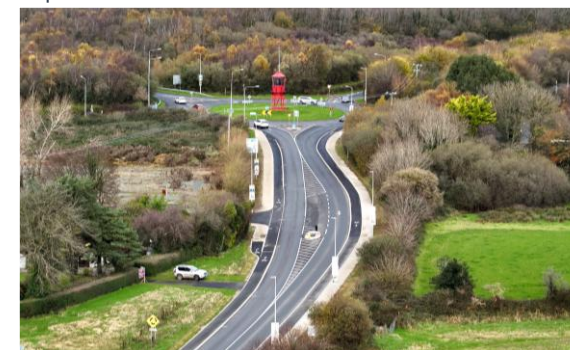
Figure 11-4: Arklow North Cycle and Pedestrian Scheme on Dublin Road. Source: WCC.
