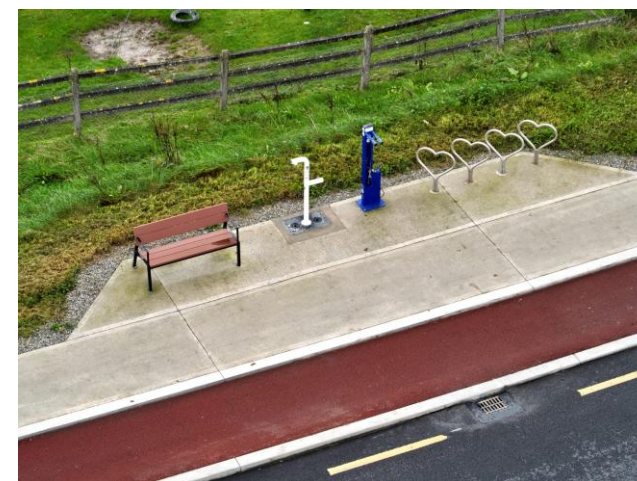
Figure 17-2: Bicycle parking, bicycle pump and a bench - delivered as part of the Arklow South Cycle and Pedestrian Scheme. Source: WCC.
