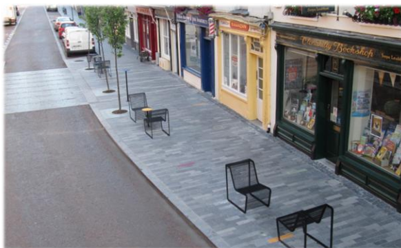
Figure 12-13: Widened area of pavement with seating and street trees in Clonakilty. The extended area was previously used for parking. However, as can be seen in the distance extensive parking bays have been retained along the street to provide loading, short-term and disabled parking bays. Source: DMURS.
