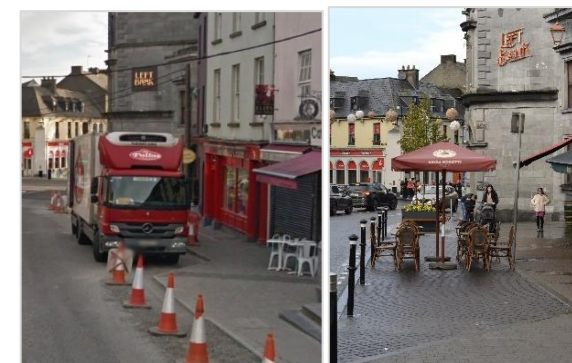
Figure 16-6: A loading bay in Kilkenny was upgraded by designing it at-grade with the footpath so it could revert to pedestrian and 'spill-out' space for local businesses when not used (after on the right). Source: DBFL.
